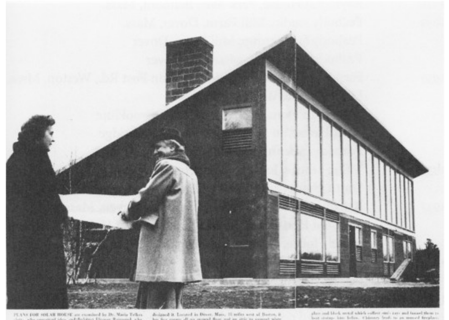
PLANS FOR SOLAR HOUSE are examined by Dr. Maria Telkes (left), who conceived idea, and architect Eleanor Raymond, who designed it. Located in Dover, Mass., 11 miles west of Boston, it has five rooms all on ground floor and an attic as support plate glass and black metal which collect sun's rays and transfer them to heat storage tank below. Chimney leads to an unusual fireplace.
